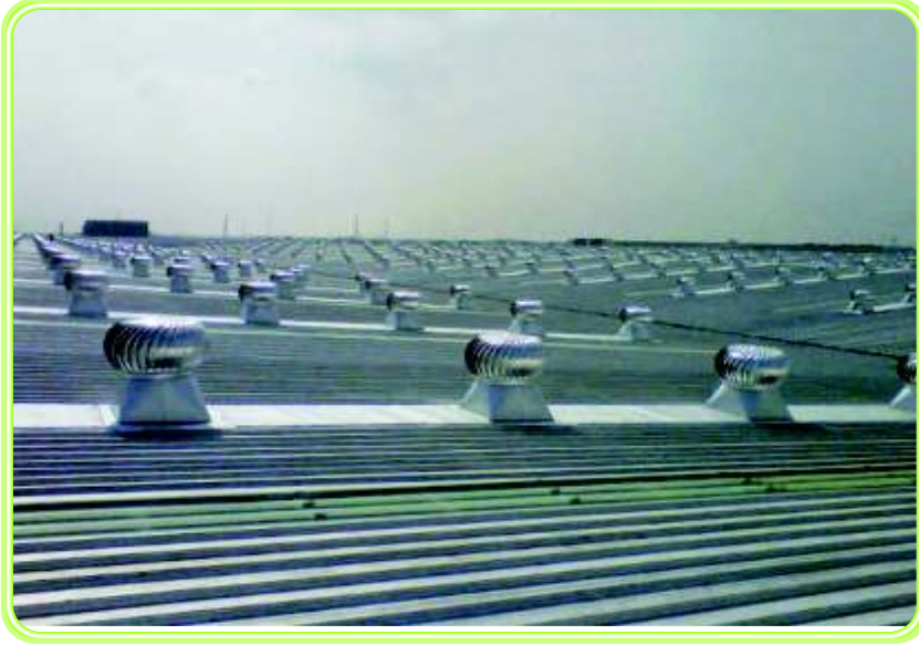
● INSTALLATION CYCLONE EXHAUST
